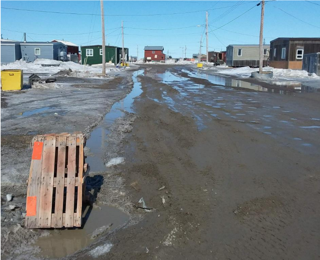
Figure 3: Example of Lack of Road-Crowning and Proper Ditching
