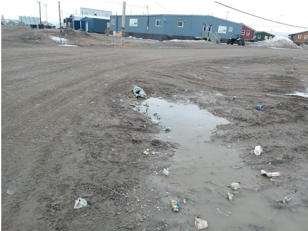
Figure 40: End of culvert at 9 th avenue and 6 th street intersection
