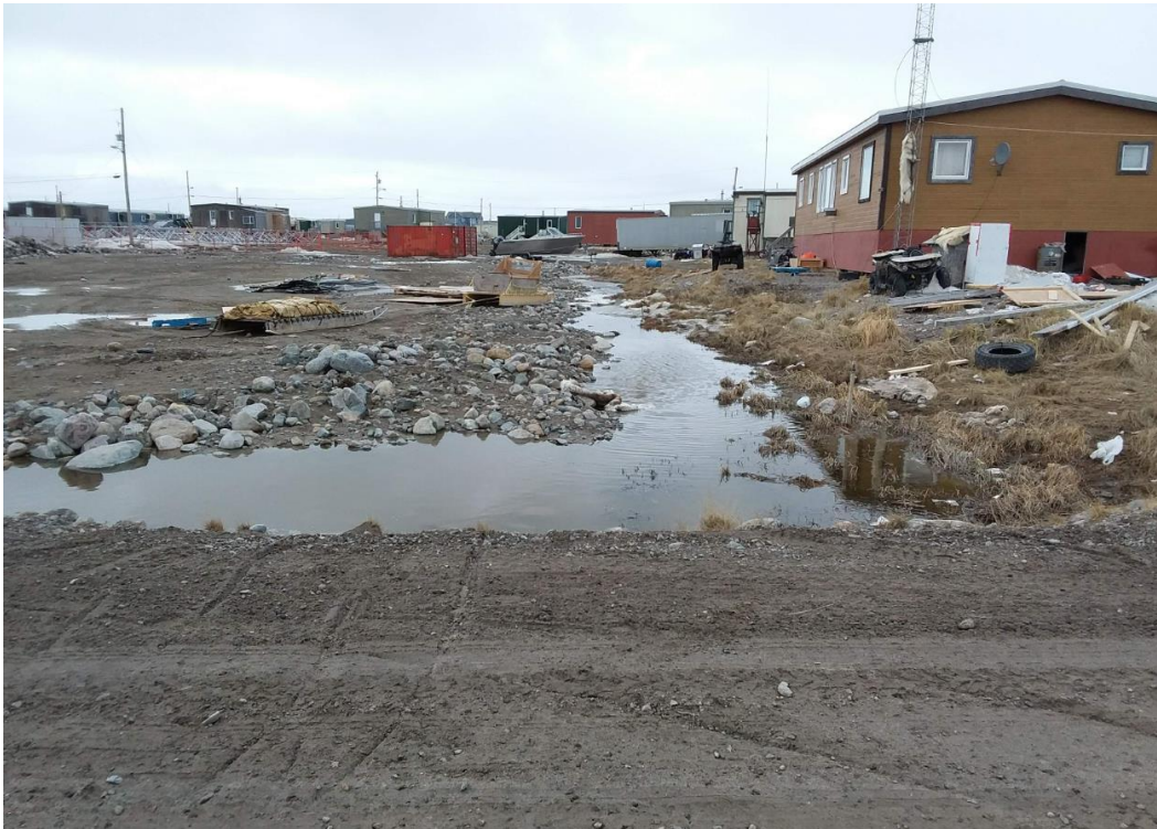
Figure 10: Standing water near new development and 11 th street
