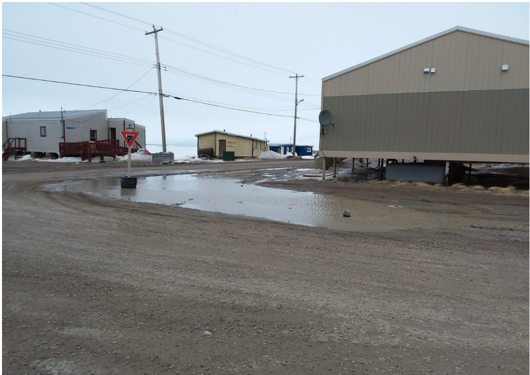
Figure 24: Water sitting at intersection of 3 rd avenue and 5 th avenue
