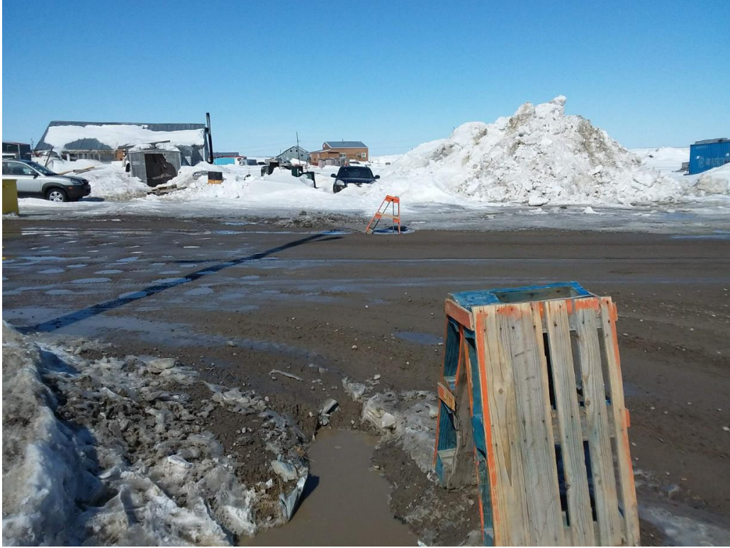
Figure 13: Culvert going north across 3 rd avenue
