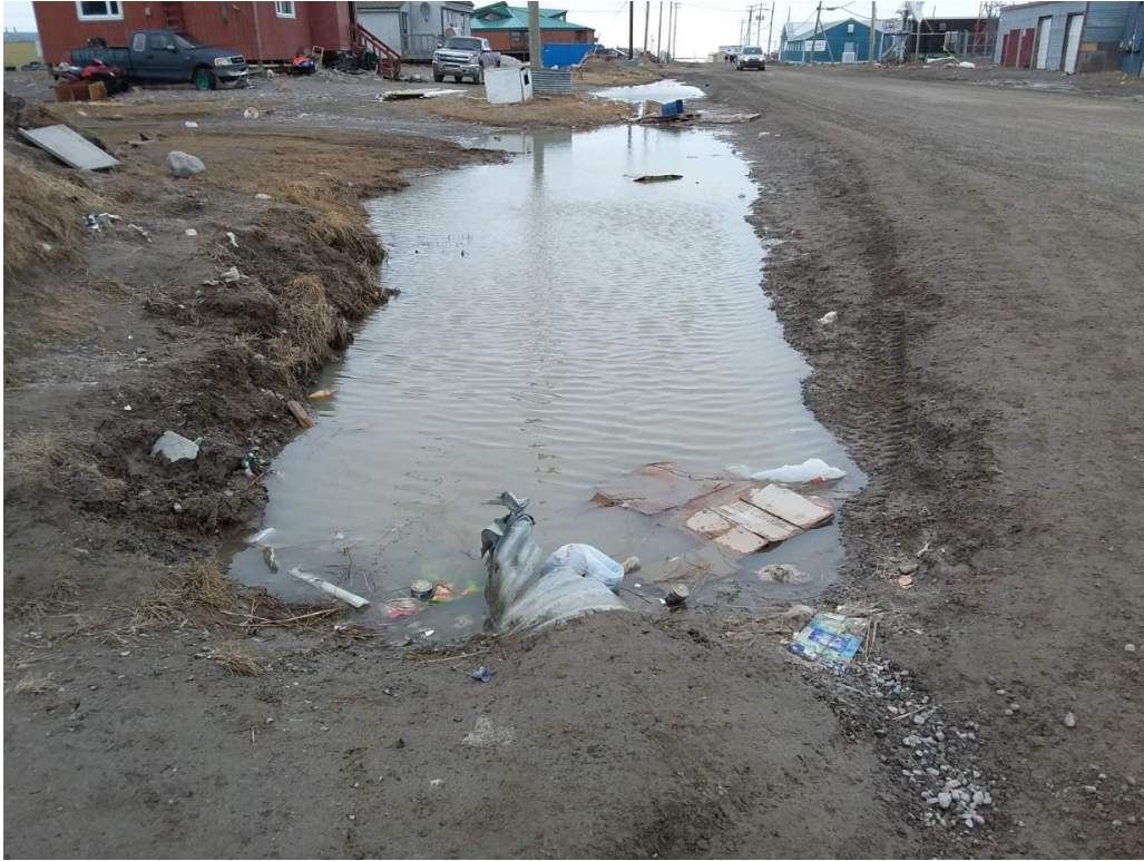
Figure 41: End of culvert at 8 th avenue and 6 th street intersection
