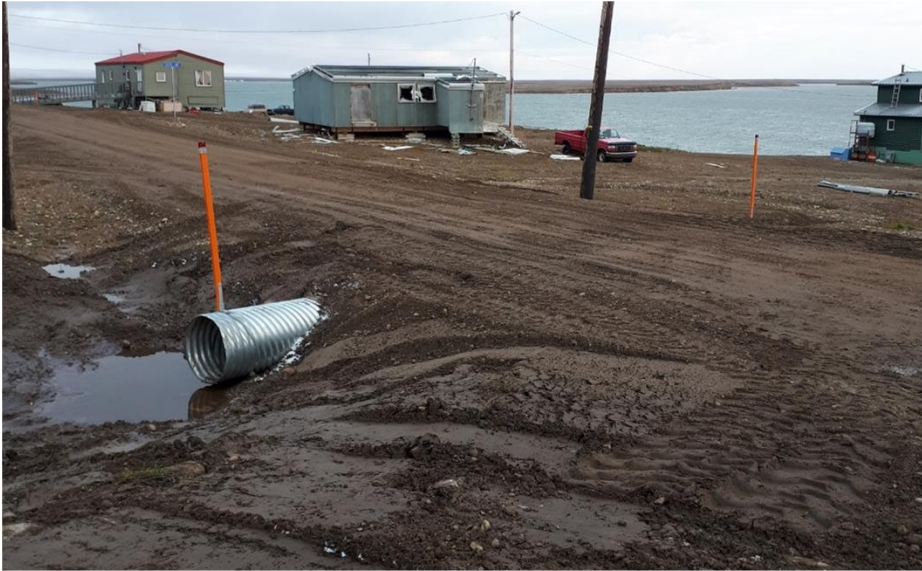
Figure 24: Example of Culvert Marker
