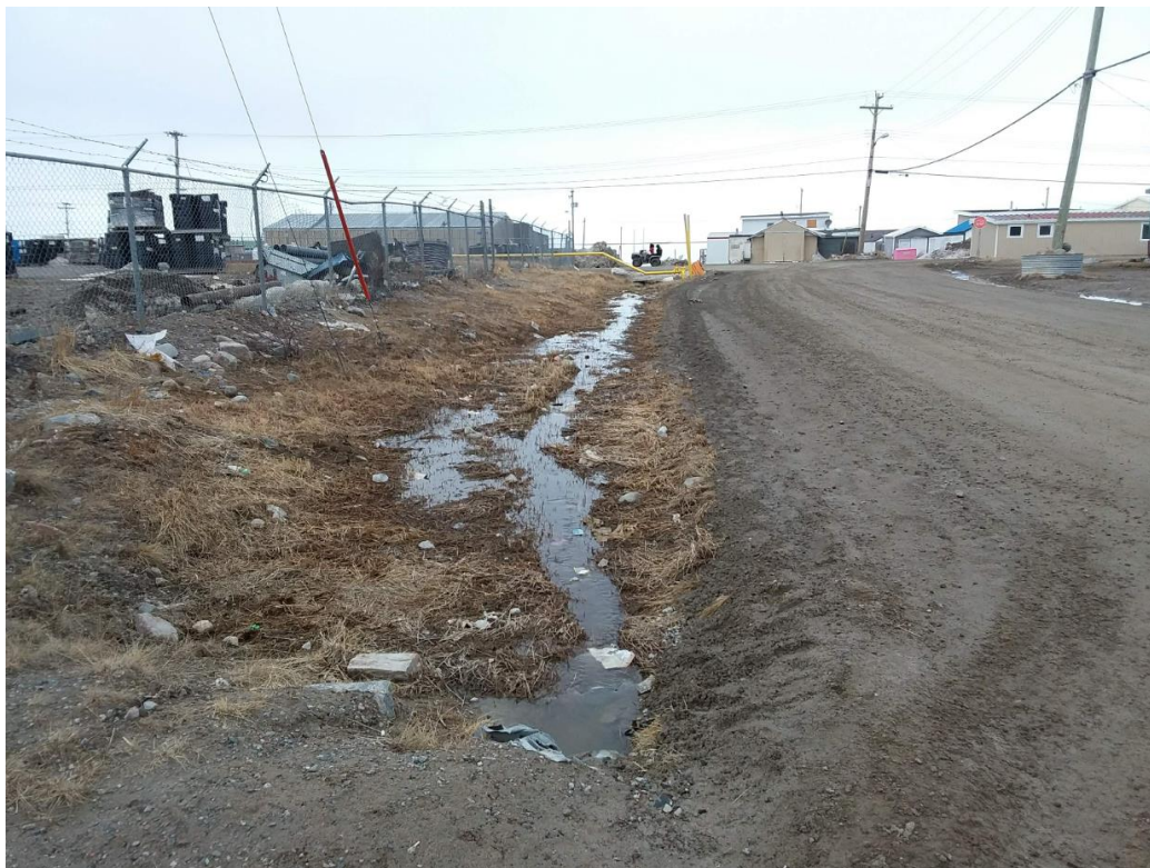
Figure 44: Ditch on west side of 6 th street looking north towards 4 th avenue intersection
