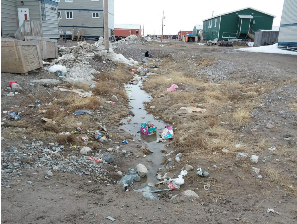
Figure 1: Ditch and end of culvert condition looking northeast
