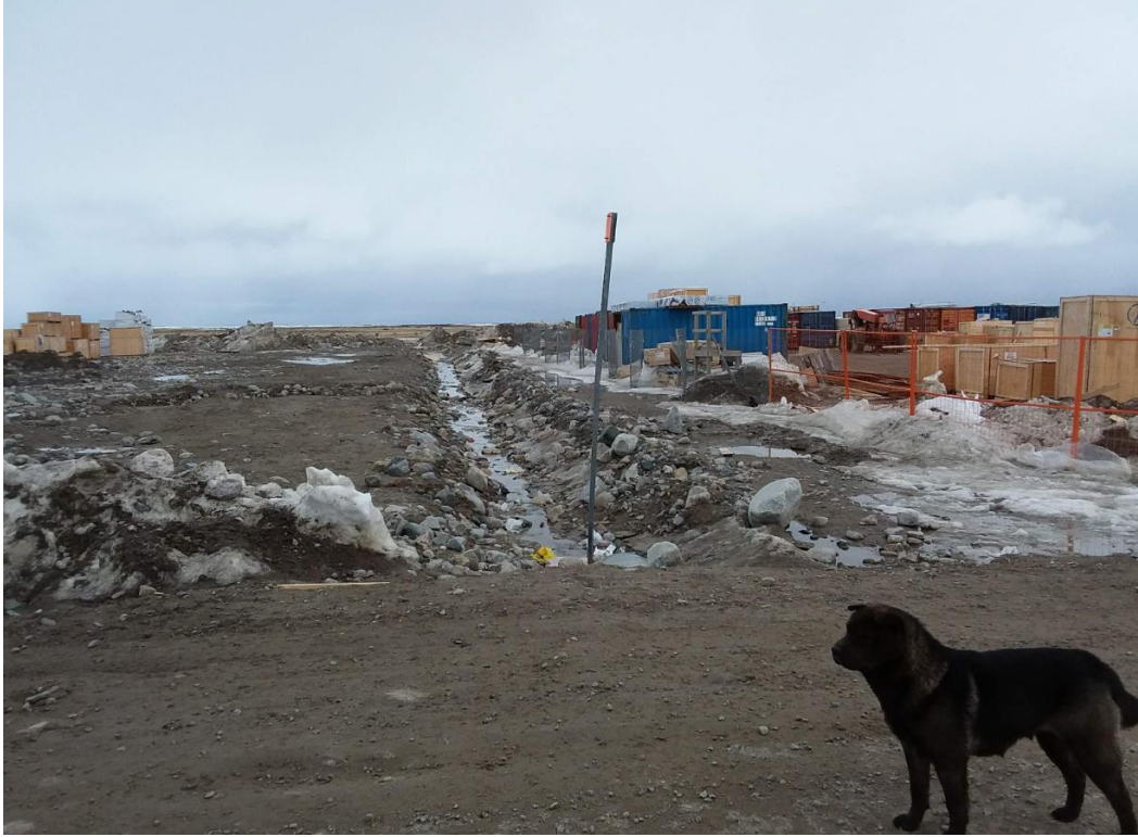
Figure 9: Looking east at drainage ditch near new development
