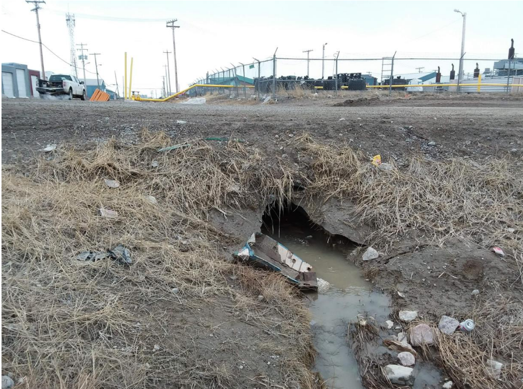
Figure 21: End of culvert at end of 6 th street
