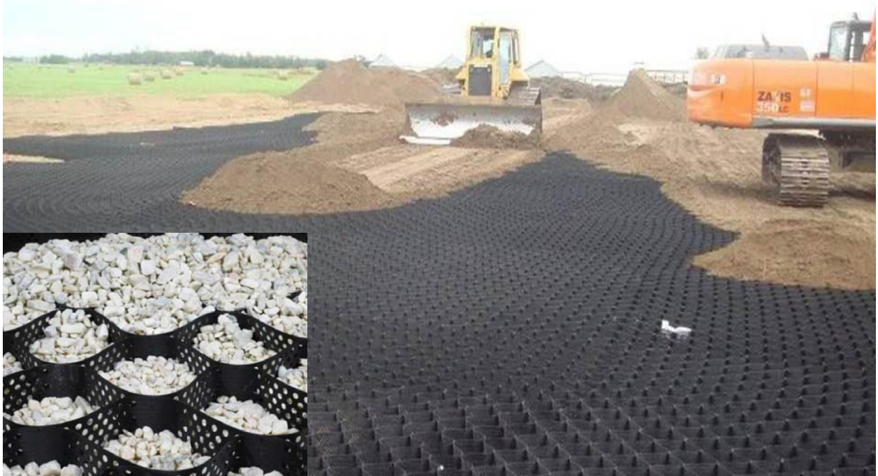
Figure F-3: Geoweb® Installation and Infilling with Aggregate
