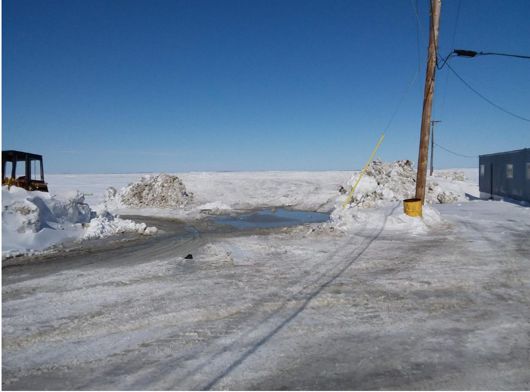
Figure 17: Snowpad location at end of 1 st avenue
