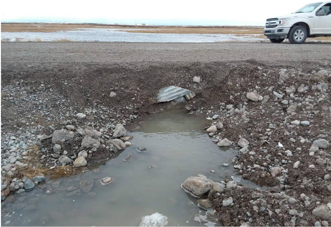
Figure 27: North end of culvert on 8 th avenue looking south
