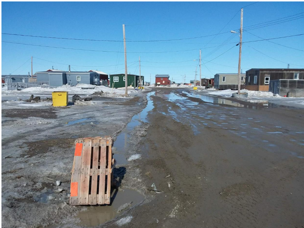
Figure 8: Looking north on 9 th street from 7 th avenue intersection
