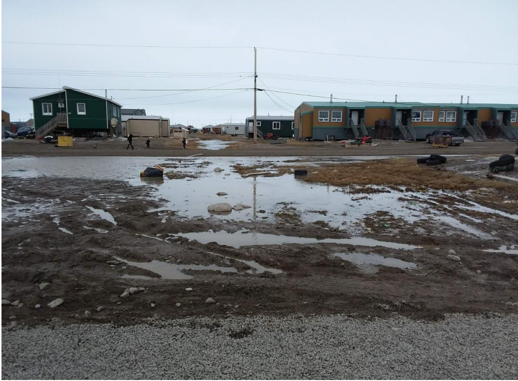
Figure 5: Condition of empty lot (looking north from photo location)
