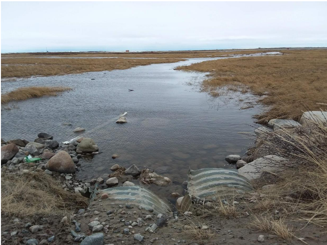
Figure 26: End of twin culverts, looking south off of 8 th avenue
