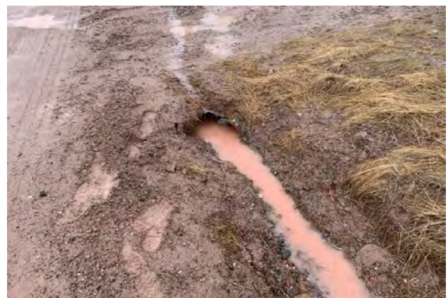
Downstream Culvert End
