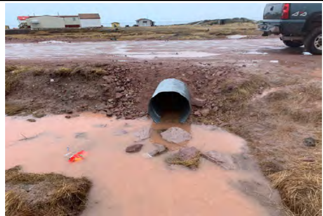
Downstream Culvert End
