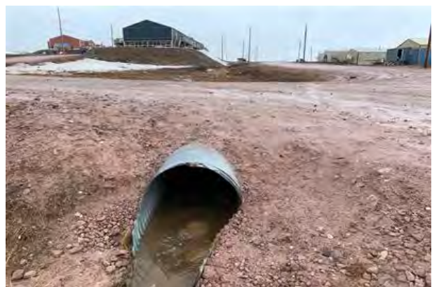
Downstream Culvert End
