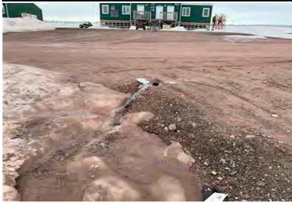
Downstream Culvert End
