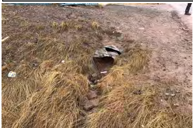
Downstream Culvert End
