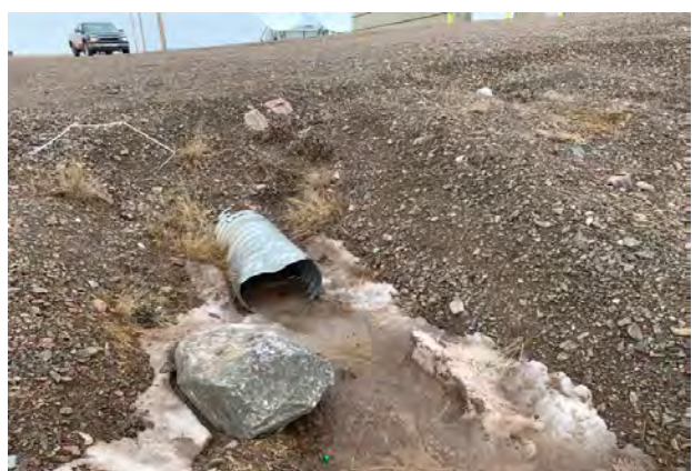
Downstream Culvert End
