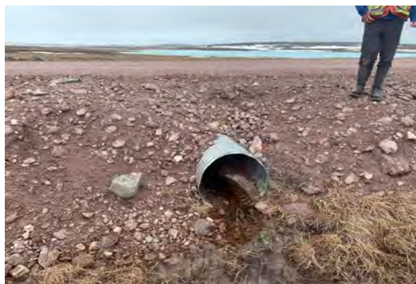
Downstream Culvert End
