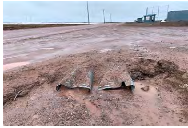
Downstream Culvert End
