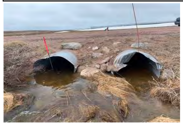
Downstream Culvert End
