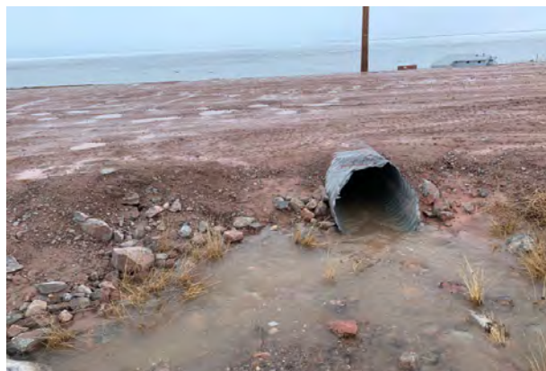
Downstream Culvert End
