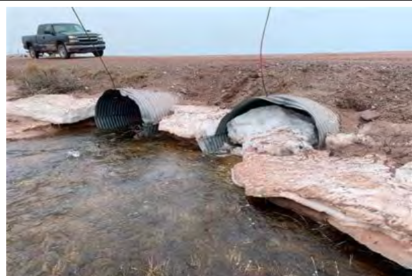
Downstream Culvert End
