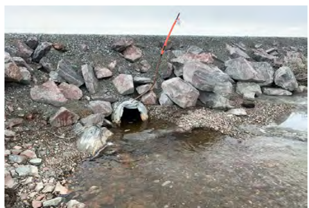
Downstream Culvert End
