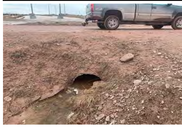
Downstream Culvert End
