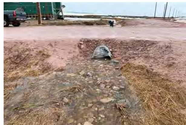
Downstream Culvert End
