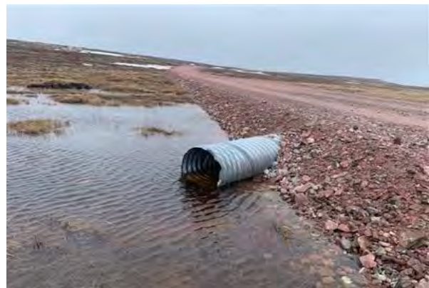
Downstream Culvert End
