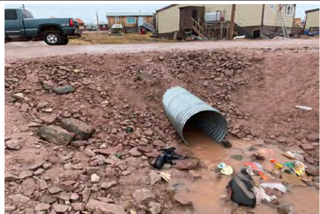
Downstream Culvert End
