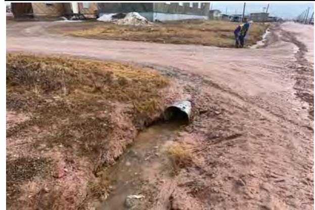
Downstream Culvert End
