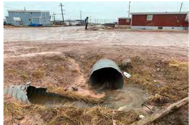
Downstream Culvert End
