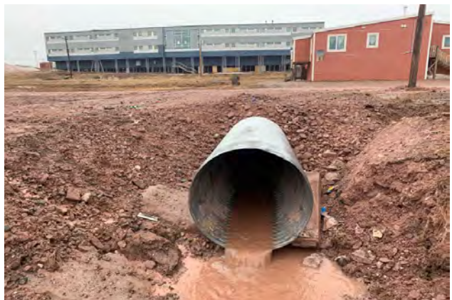
Downstream Culvert End
