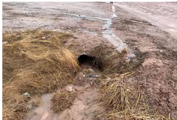
Downstream Culvert End
