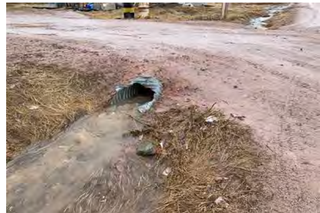
Downstream Culvert End
