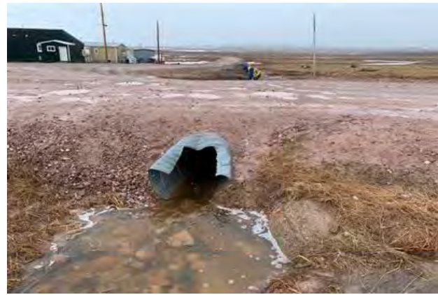
Downstream Culvert End
