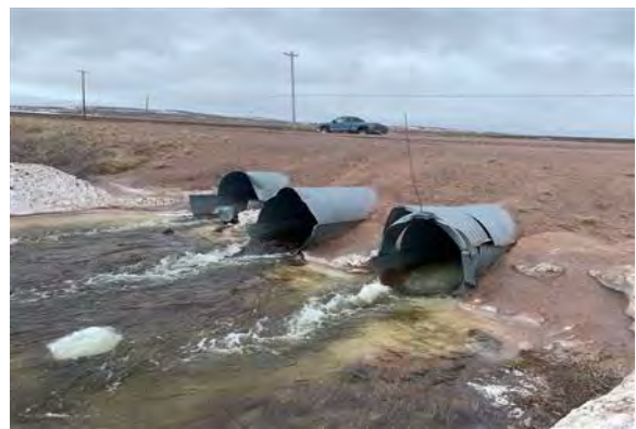
Downstream Culvert End
