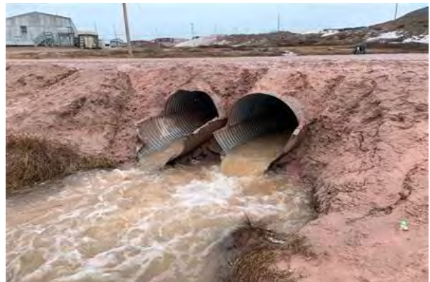
Downstream Culvert End
