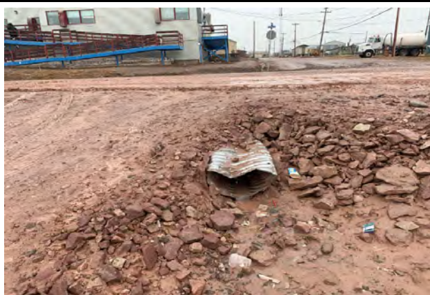
Downstream Culvert End
