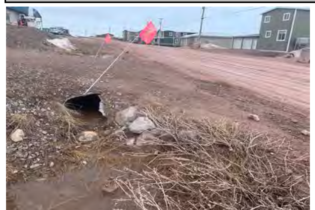
Downstream Culvert End
