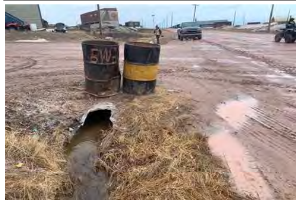
Downstream Culvert End
