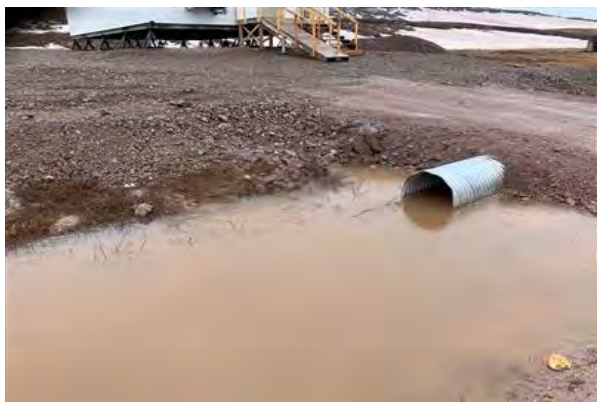
Downstream Culvert End
