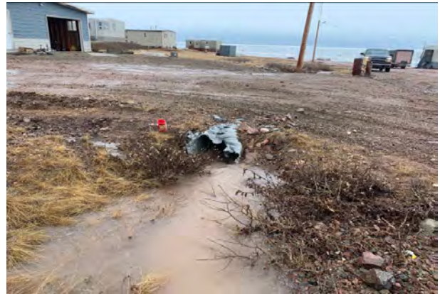
Downstream Culvert End
