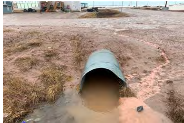
Downstream Culvert End
