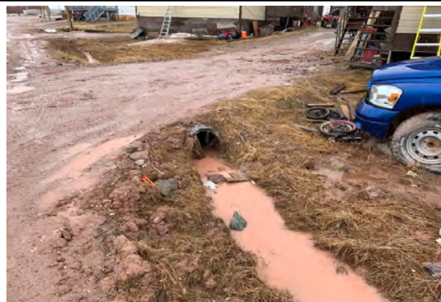
Downstream Culvert End
