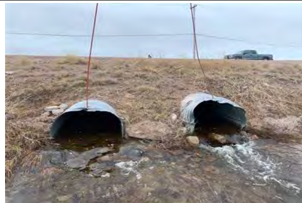
Downstream Culvert End
