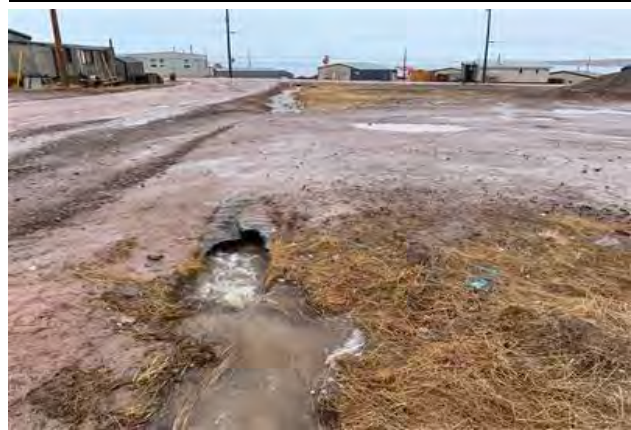
Downstream Culvert End
