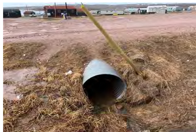
Downstream Culvert End
