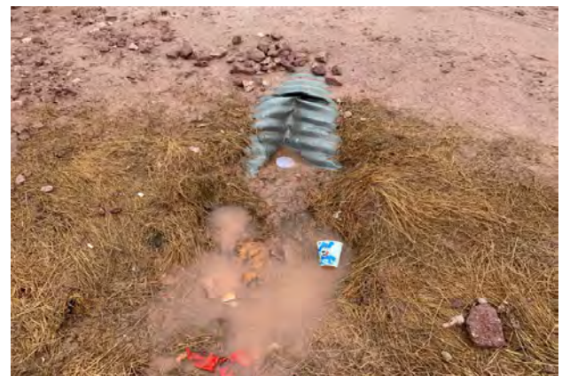
Downstream Culvert End
