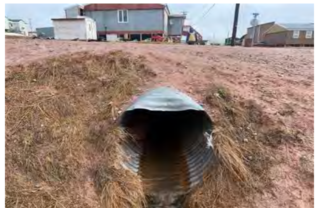
Downstream Culvert End
