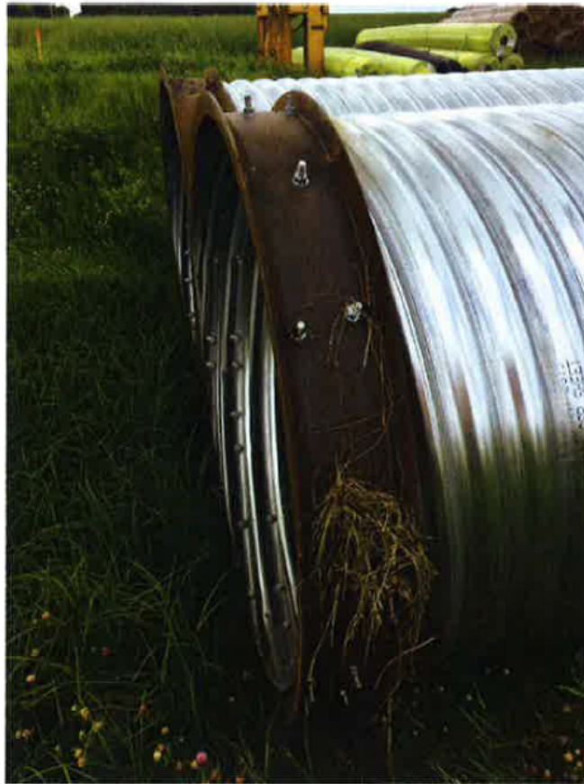
Figure 17 Example of culvert end treatment (See Clause 5.6.4.8. )
