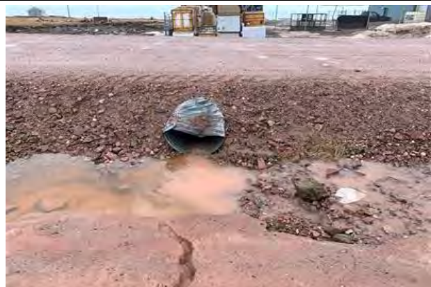
Downstream Culvert End
