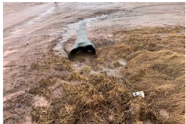
Downstream Culvert End
