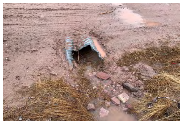
Downstream Culvert End
