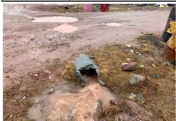
Downstream Culvert End
