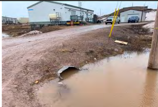
Downstream Culvert End
