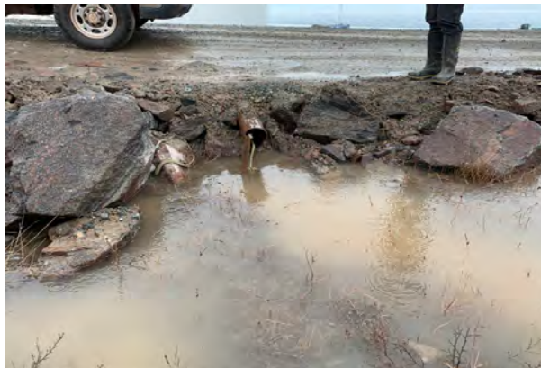
Downstream Culvert End
