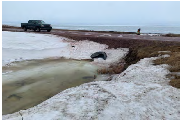
Downstream Culvert End
