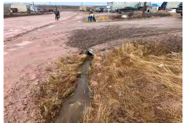
Downstream Culvert End
