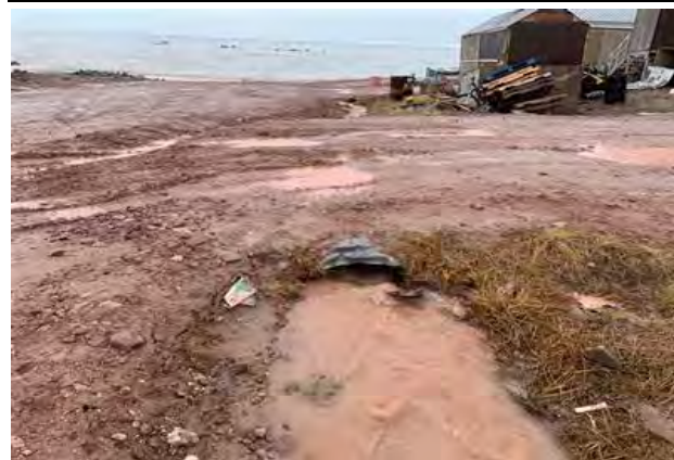
Downstream Culvert End
