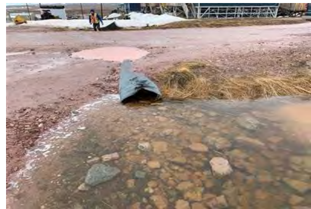
Downstream Culvert End
