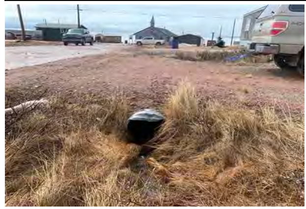
Downstream Culvert End
