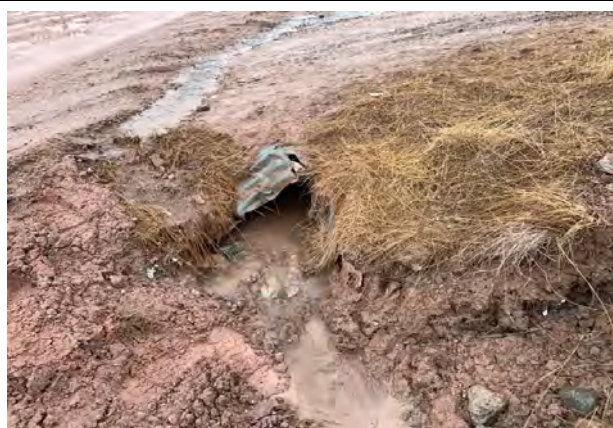
Downstream Culvert End
