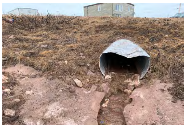
Downstream Culvert End
