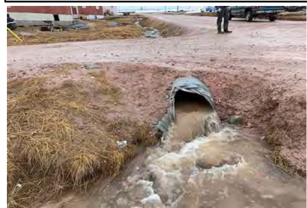
Downstream Culvert End
