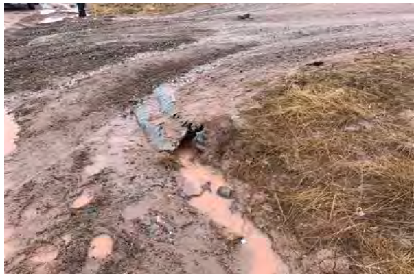
Downstream Culvert End
