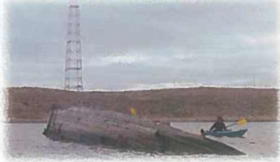
FIGURE 6 THE LORAN TOWER
