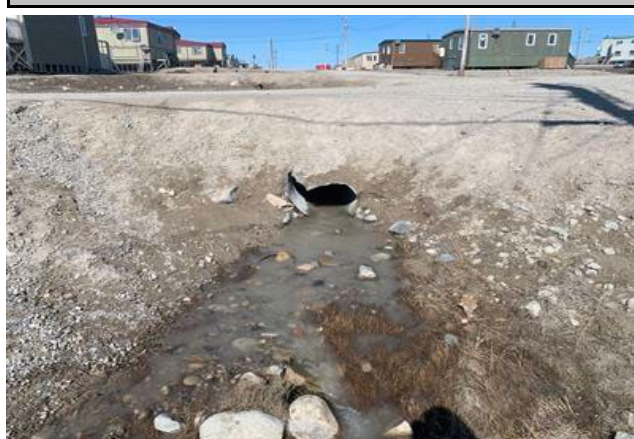
Downstream Culvert End
