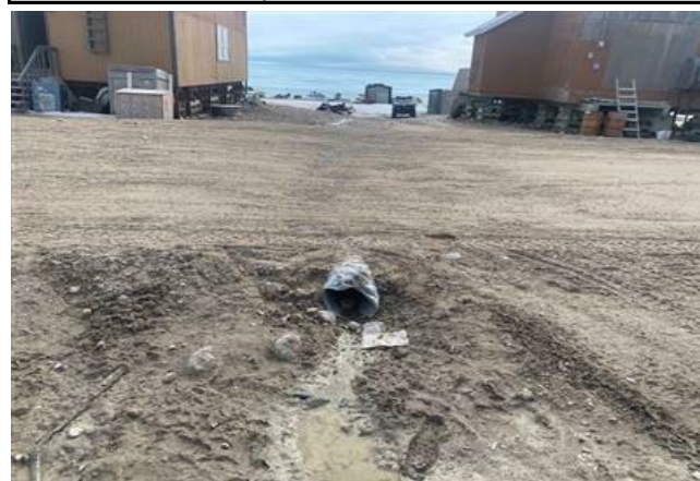
Downstream Culvert End
