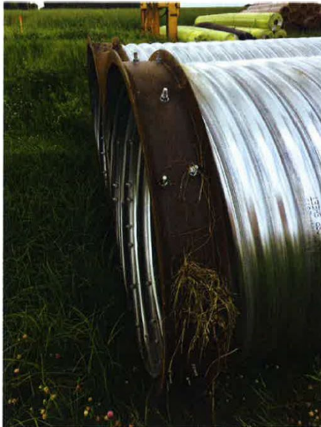
Figure 17 Example of culvert end treatment (See Clause 5.6.4.8. )
