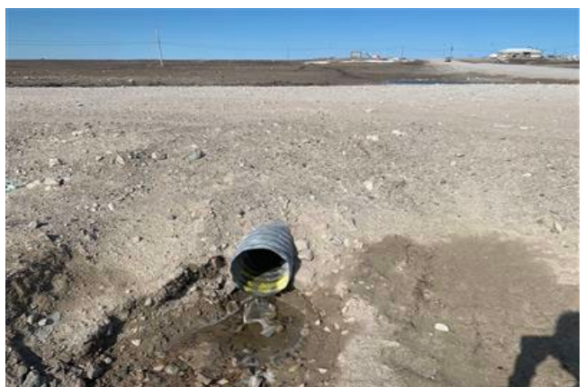
Downstream Culvert End
