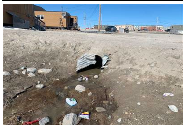
Downstream Culvert End
