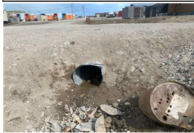
Downstream Culvert End
