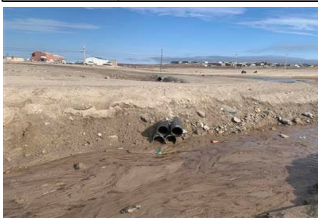
Downstream Culvert End
