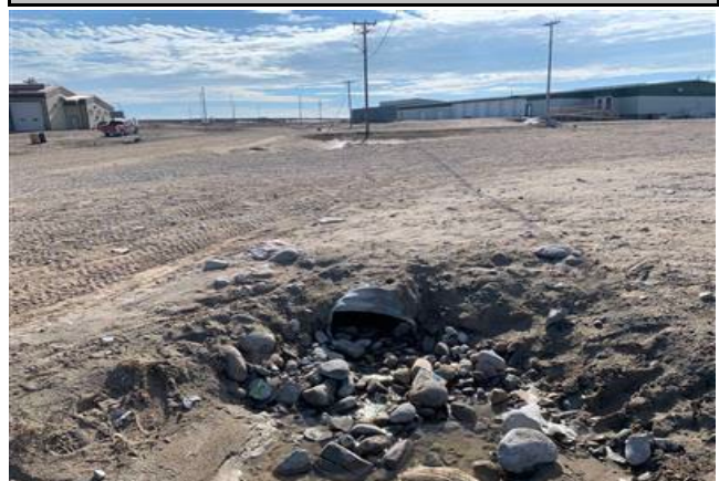
Downstream Culvert End
