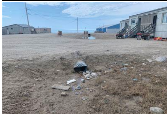
Downstream Culvert End
