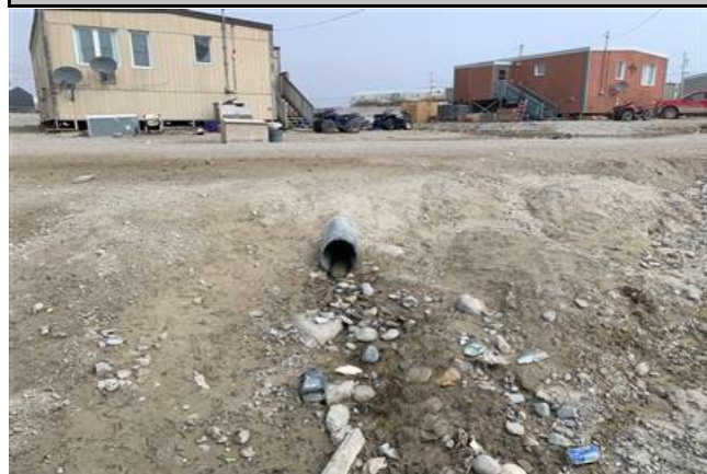
Downstream Culvert End
