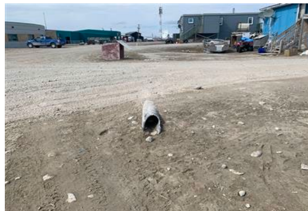
Downstream Culvert End
