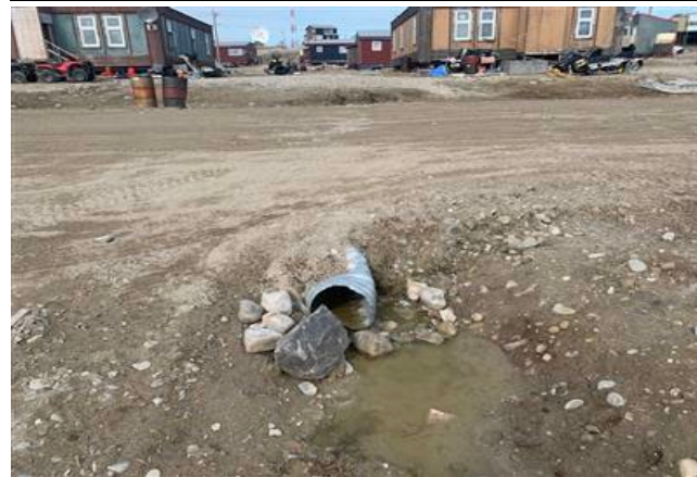
Downstream Culvert End
