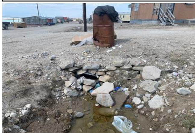
Downstream Culvert End
