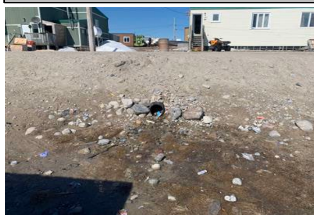
Downstream Culvert End
