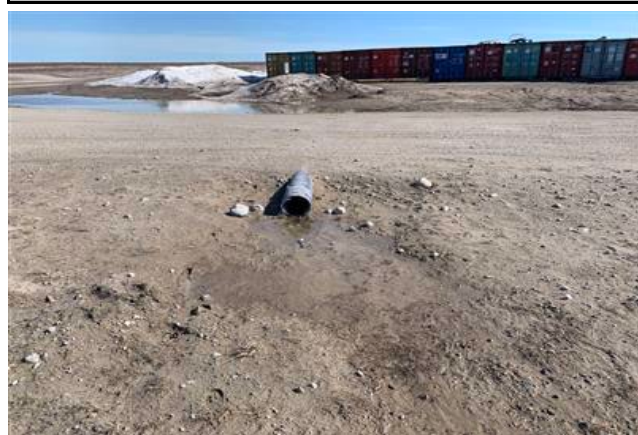
Downstream Culvert End
