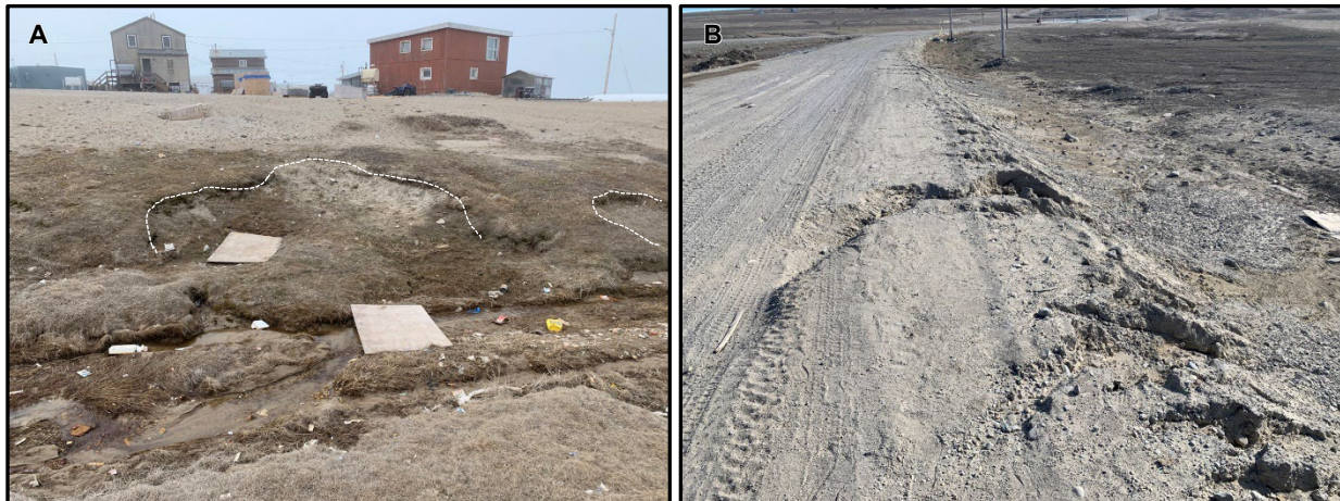
Figure 4-6 Examples of Soil Surface Erosion Observed Within the Existing Townsite. A) Erosion Scars Along the Gully that Crosses the Old Townsite (identified as white dash lines). B) Embankment Rill Erosion (IDPA #5).
