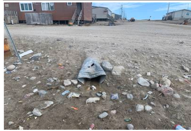
Downstream Culvert End
