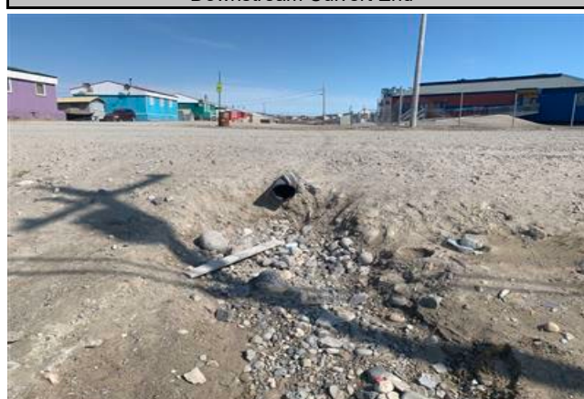
Downstream Culvert End
