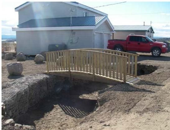
Figure 36: Properly installed culverts and footbridges ensure adequate drainage through the subdivision.
