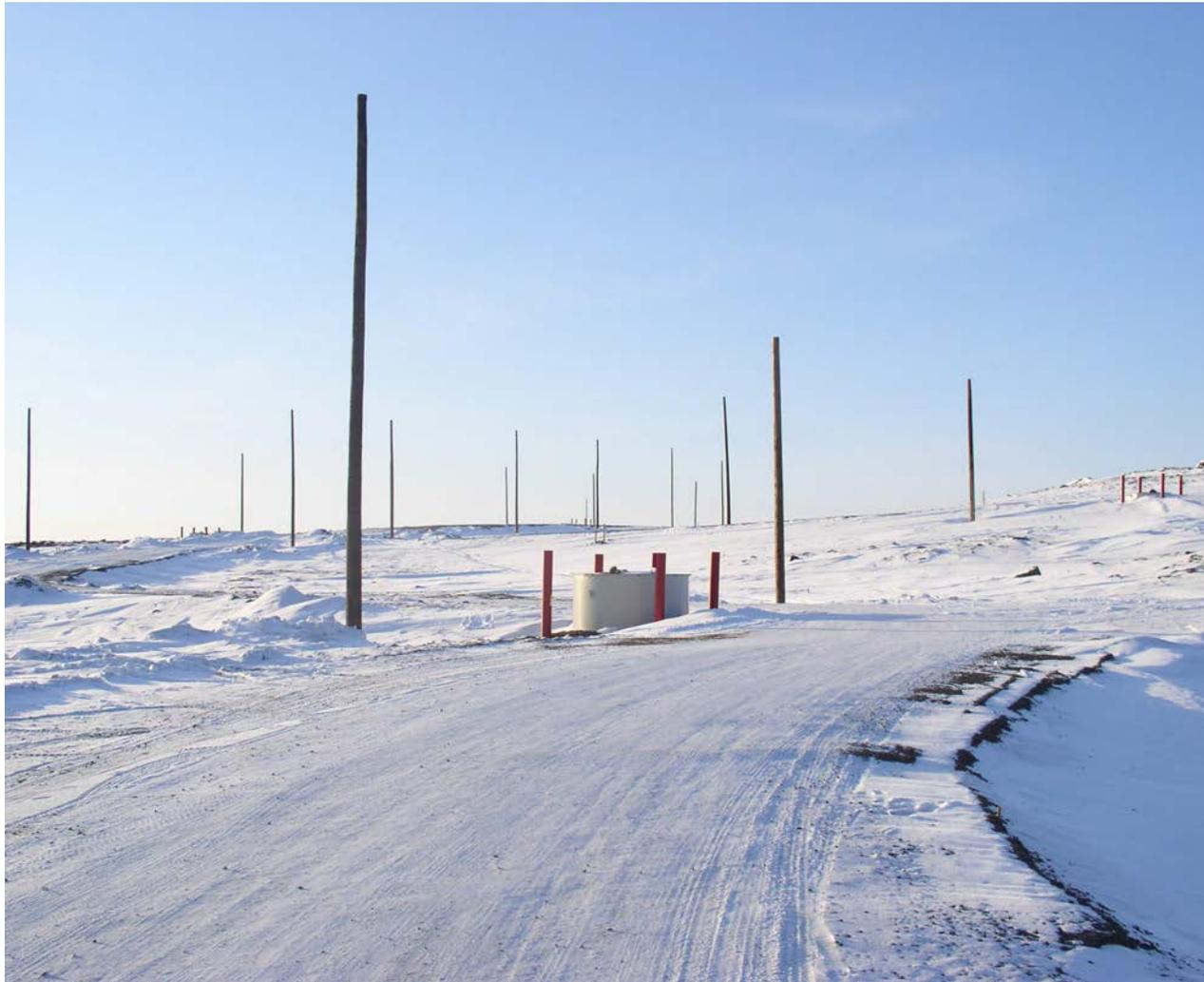
*Figure 51: Power poles and piped municipal services are typically installed in the road right-of-way prior to construction of housing and other uses.*
