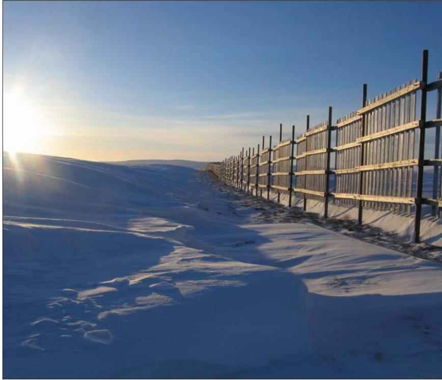
Figure 49: Snow fence with resulting drift zone.
