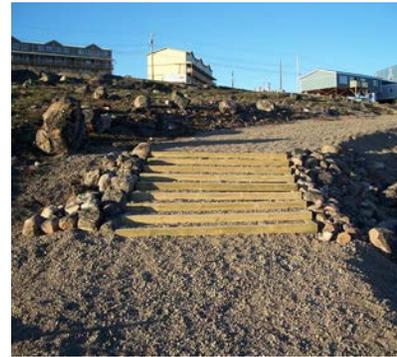
Figure 37: Small rocks can be used to accentuate the edges of walking trails. In steeper trail sections, it may be appropriate to build stairs to enhance the walking experience and prevent erosion.
