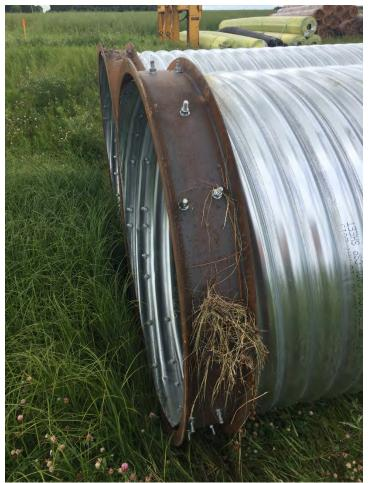
Photo 1: Example Culvert End Stiffener
