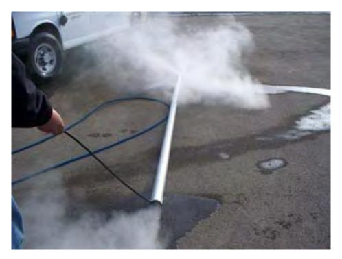
Culverts are subject to freezing during winter and spring. During winter, ground water can continuously feed streams which either flow through culverts or over roadways causing icing. During spring breakup, daytime melting must be carried through culverts.
