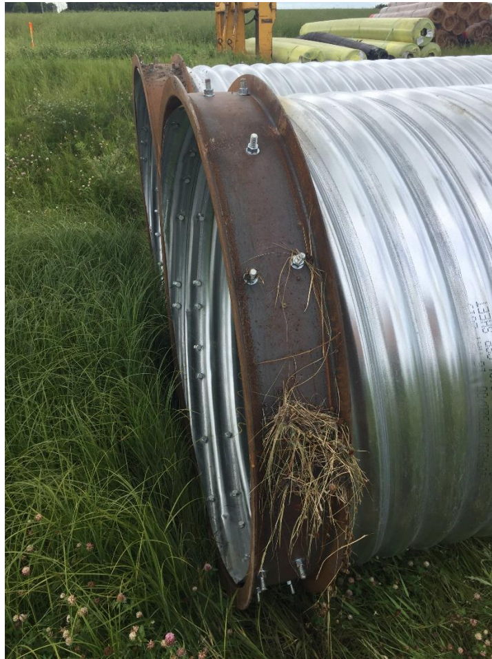
Photo 1: Example Culvert End Stiffener
