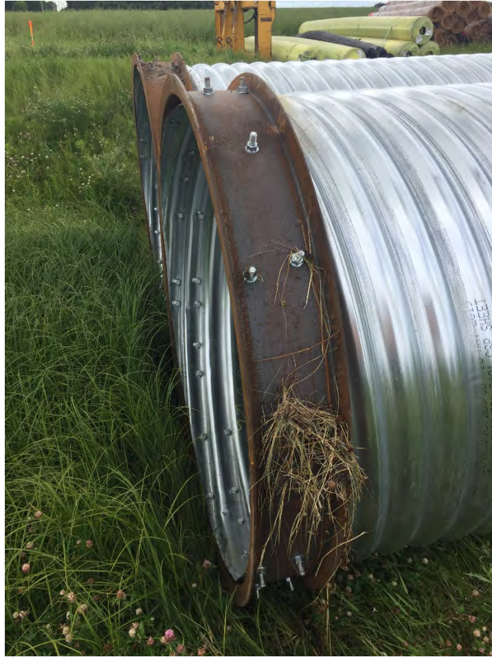
Photo 1: Example Culvert End Stiffener
