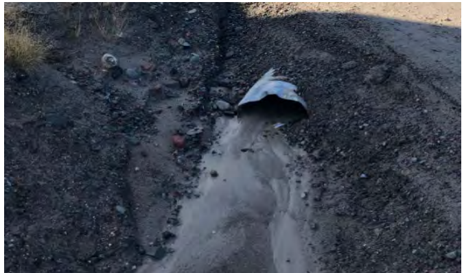
Downstream Culvert End
