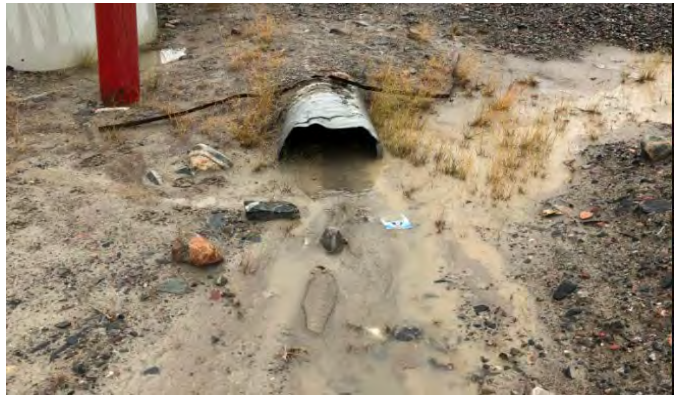
Downstream Culvert End
