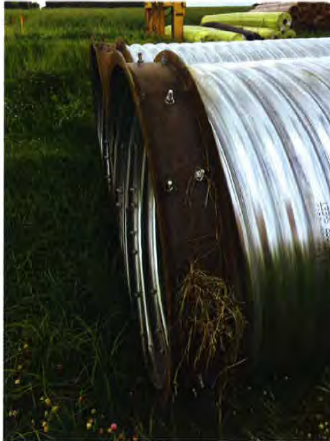
Figure 17 Example of culvert end treatment (See Clause 5.6.4.8. )
