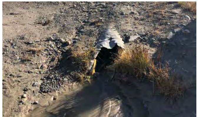
Downstream Culvert End
