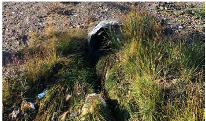
Downstream Culvert End
