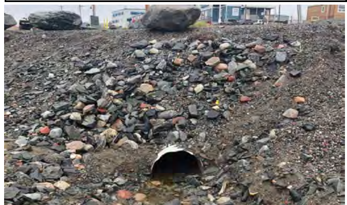
Downstream Culvert End
