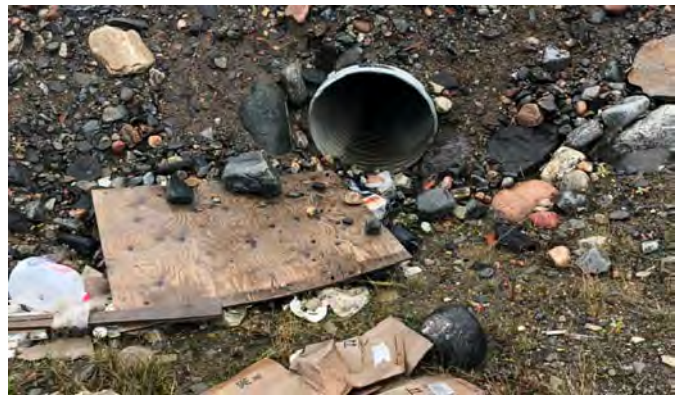
Downstream Culvert End
