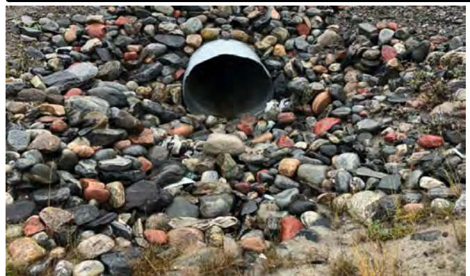
Downstream Culvert End
