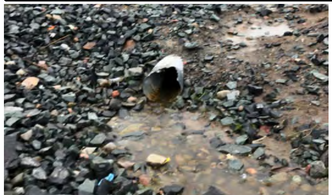
Downstream Culvert End
