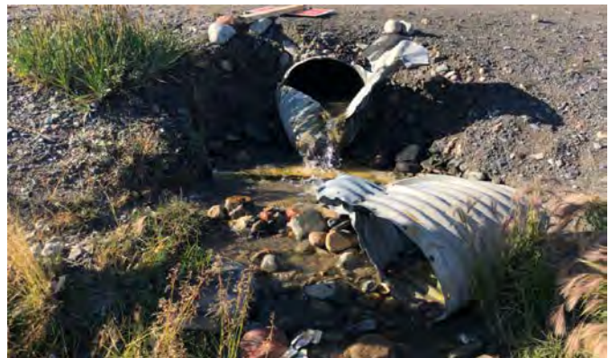
Downstream Culvert End
