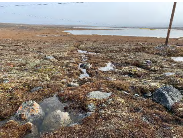
Photo 17: Ice wedge north of Block 10. Water flows within.
