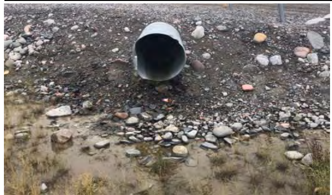
Downstream Culvert End
