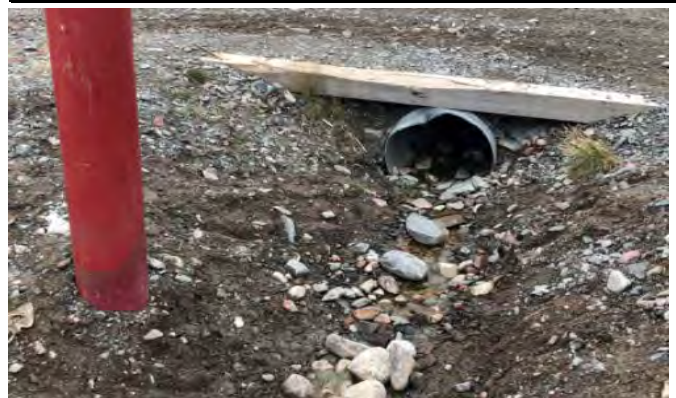
Downstream Culvert End
