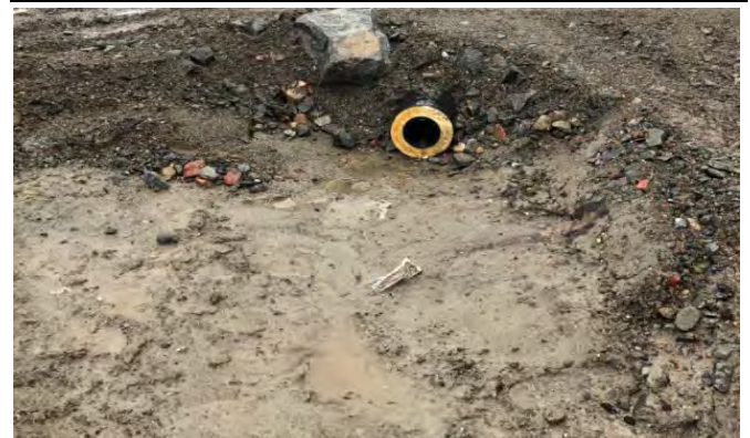
Downstream Culvert End
