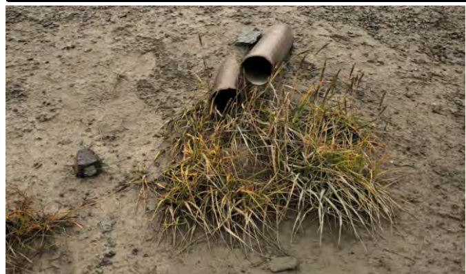
Downstream Culvert End
