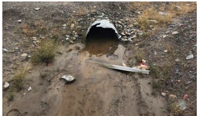
Downstream Culvert End
