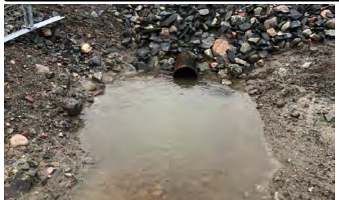
Downstream Culvert End
