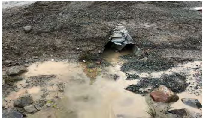
Downstream Culvert End
