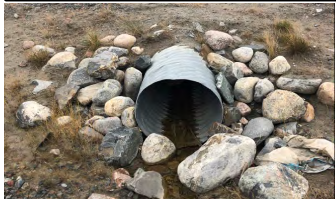
Downstream Culvert End
