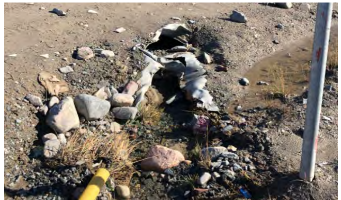
Downstream Culvert End
