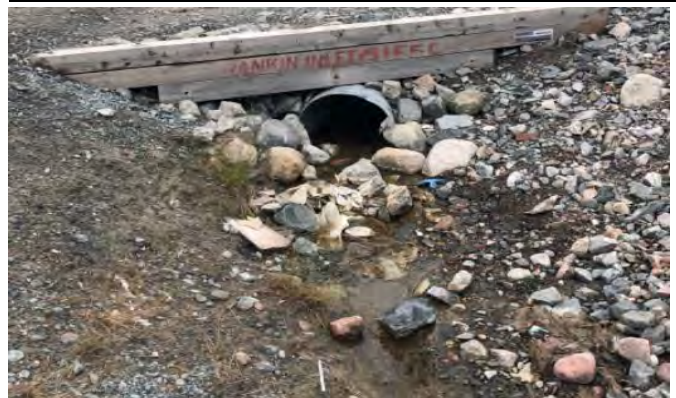
Downstream Culvert End
