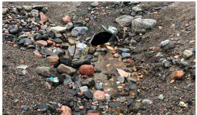
Downstream Culvert End
