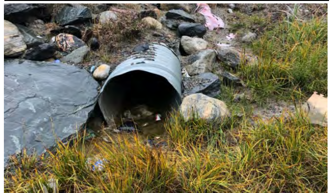
Downstream Culvert End
