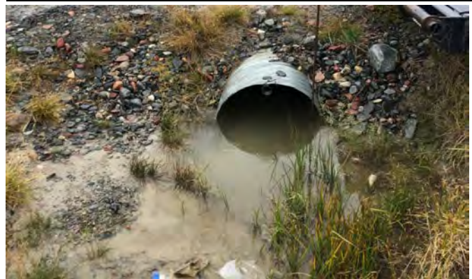
Downstream Culvert End
