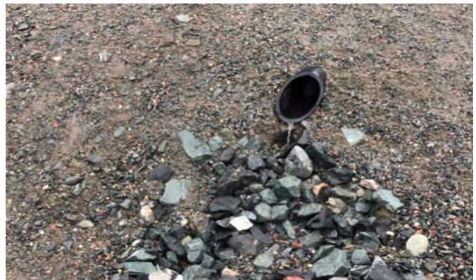
Downstream Culvert End
