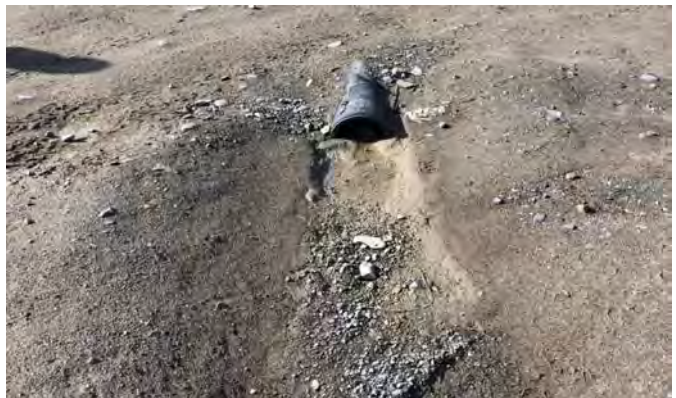
Downstream Culvert End
