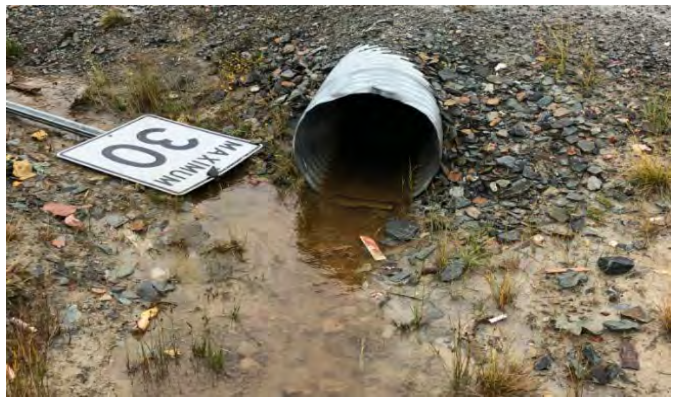
Downstream Culvert End
