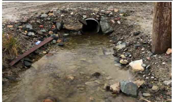
Downstream Culvert End
