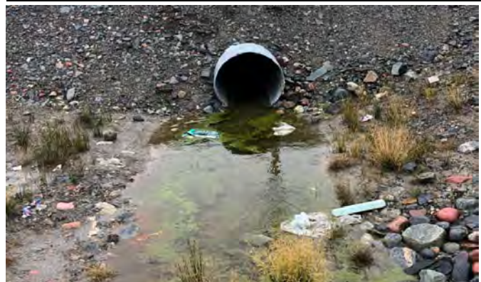
Downstream Culvert End
